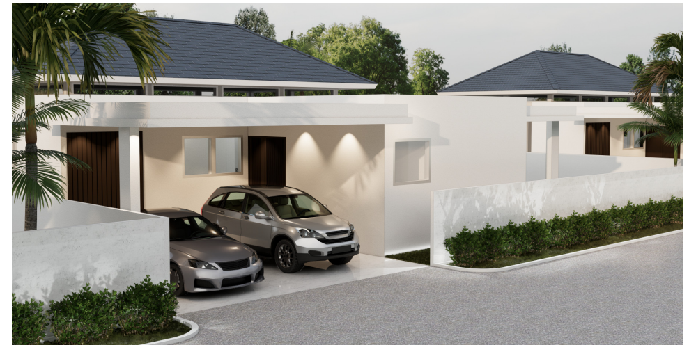
Villa seen from the road- entrance
